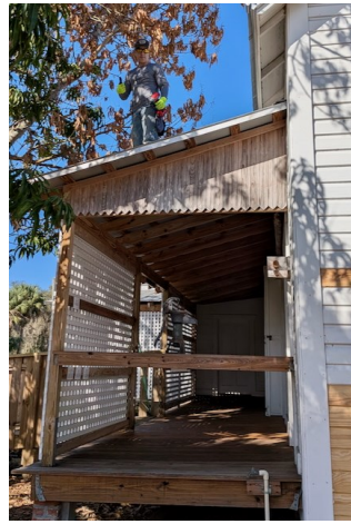
H. Rescrewing south porch
